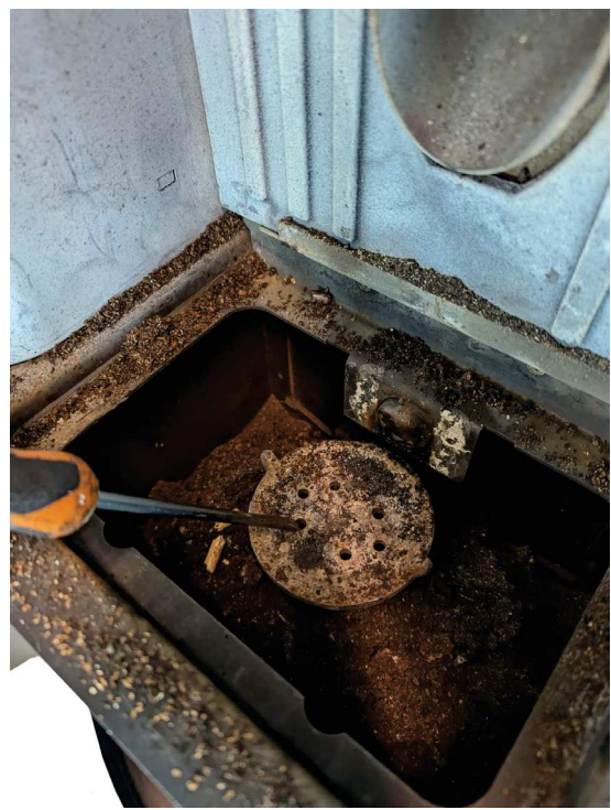
Fig. 37 - Burning pot cleaning
