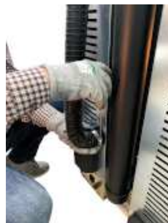
Fig. 45 - Insert combustion air pipe
