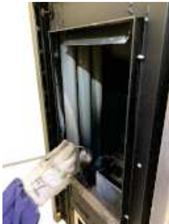
Fig. 77 - Clean with pipe cleaner
