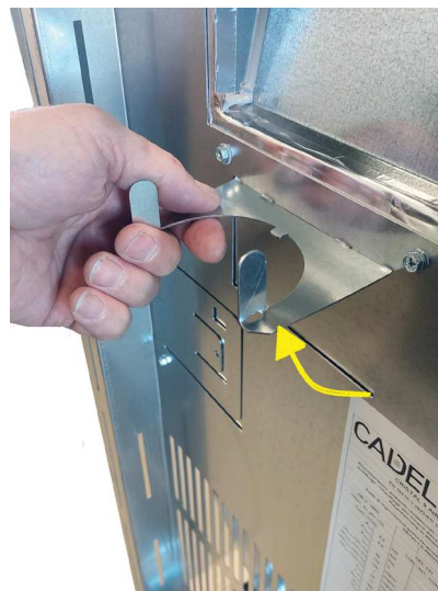
Fig. 39 - Fold the tabs
