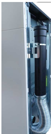
Fig. 57 - Block pipe d.80 mm
