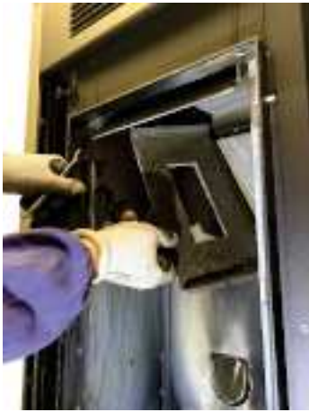
Fig. 74 - Remove the head of the firebox 2
