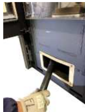
Fig. 69 - Vacuum out the ash
