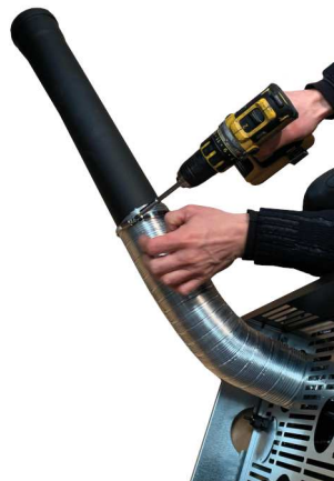
Fig. 55 - Connect pipe d.80 mm
