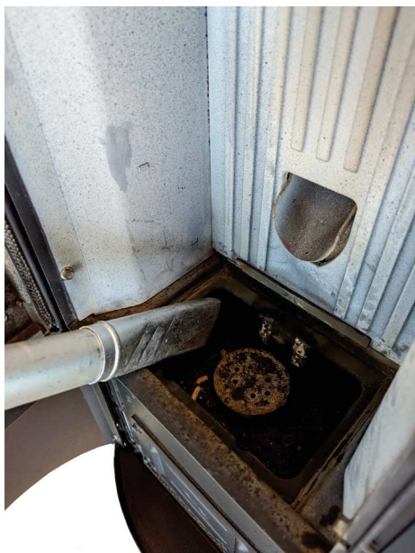
Fig. 40 - Burning pot box cleaning
