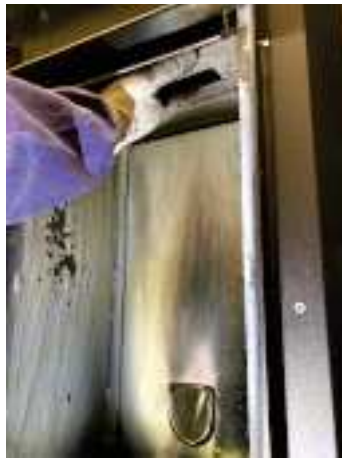
Fig. 91 - Remove the head of the firebox 1
