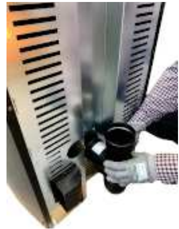
Fig. 56 - Connect the Tee fitting
