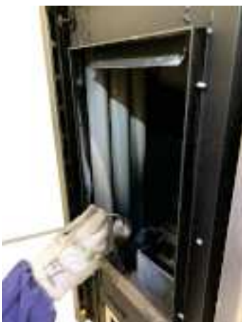
Fig. 95 - Clean with pipe cleaner
