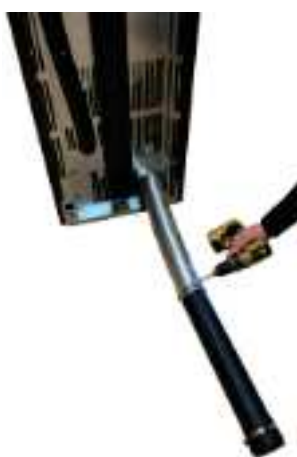
Fig. 74 - Connect pipe d.80 mm
