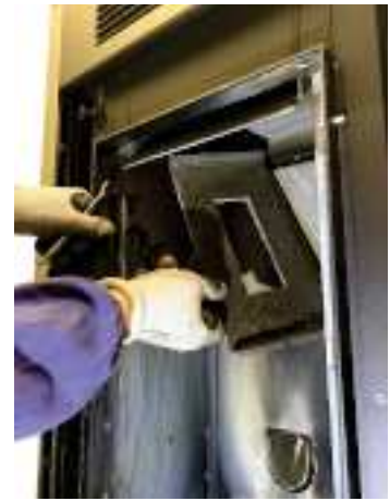
Fig. 92 - Remove the head of the firebox 2
