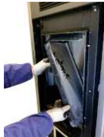
Fig. 94 - Remove the side walls
