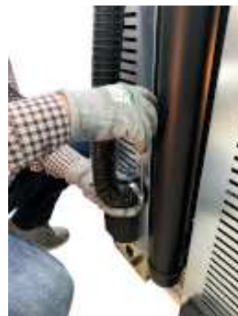
Fig. 64 - Insert combustion air pipe
