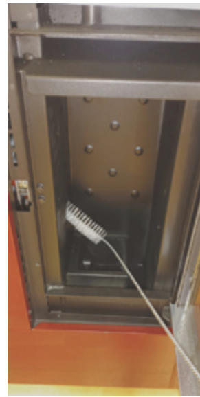
Fig. 35 - Cleaning with a brush
