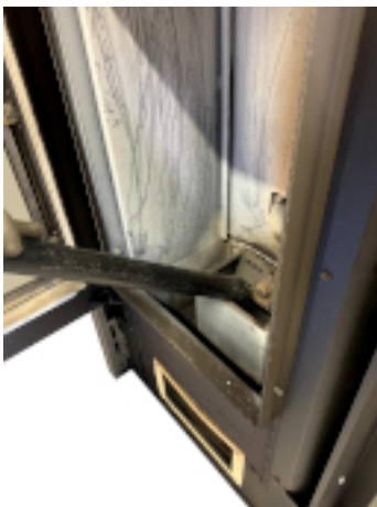
Fig. 35 - Burning pot box cleaning
